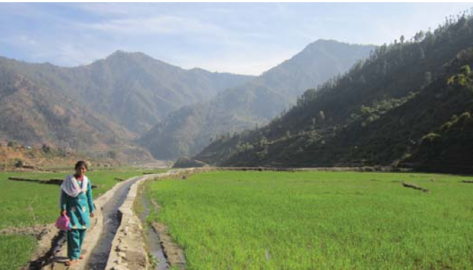
Concrete-lined canal in the hills
