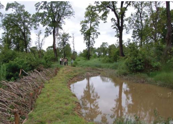
Canal of a SSIS with brushwood dam
